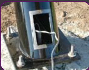
Sign during various stages of installation
