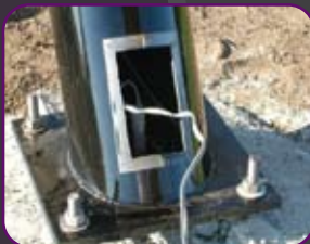
Sign during various stages of installation
