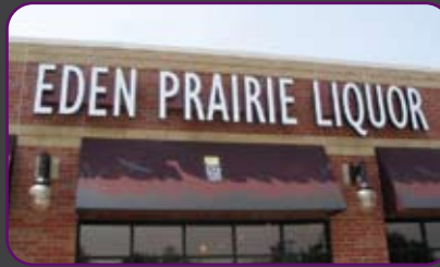
Internally lit channel letters and awning graphics
